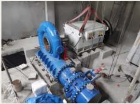
ERECTION AT JEULI GAD, NEPAL 1 x 1 MW, Horizontal Francis
