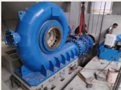
LOWER CHHOTE KHOLA, NEPAL 2 x 0.5 MW, 2 Jet Horizontal Pelton
